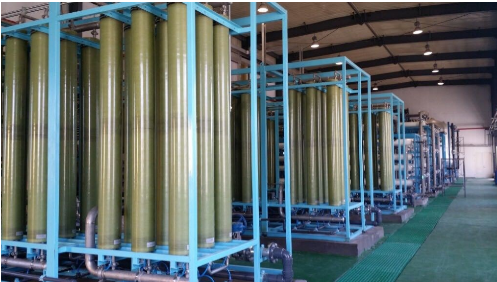
Membrane Skids with Double Length STRO modules
